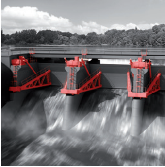
Hydro-electric power stations
